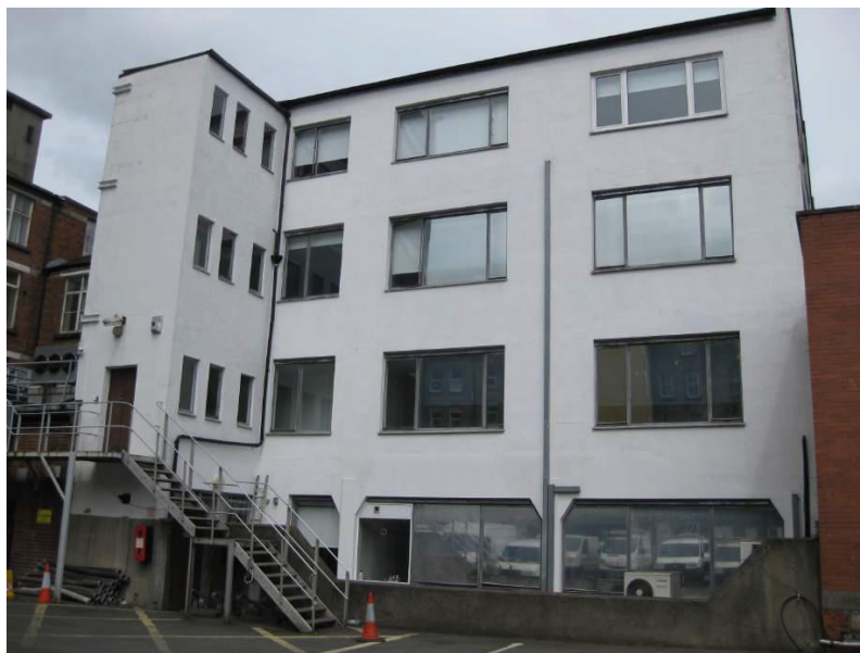
Rear elevation (Niamh Marnham, 2015)
