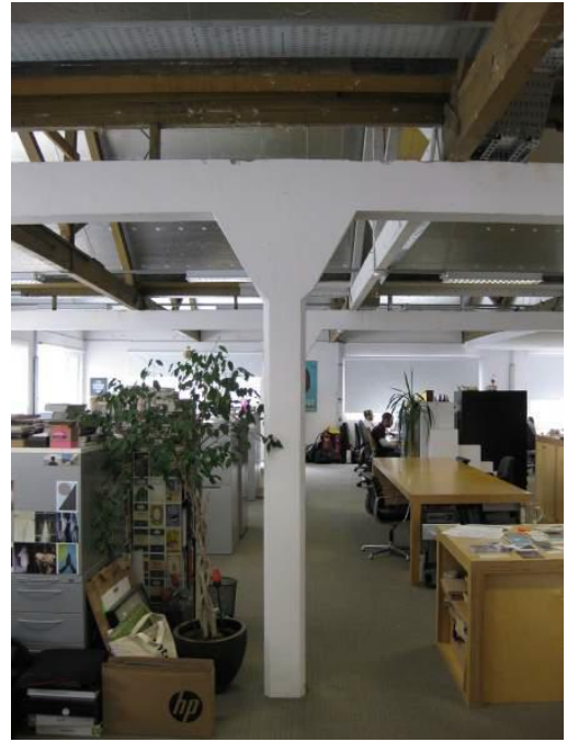
Interior spaces with exposed Hennebique concrete structure
