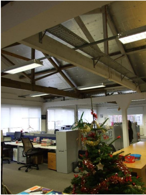
Interior spaces with exposed Hennebique concrete structure
